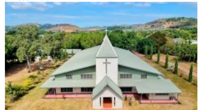
An aerial view of the St Charles Lwanga Church and Parish grounds.
